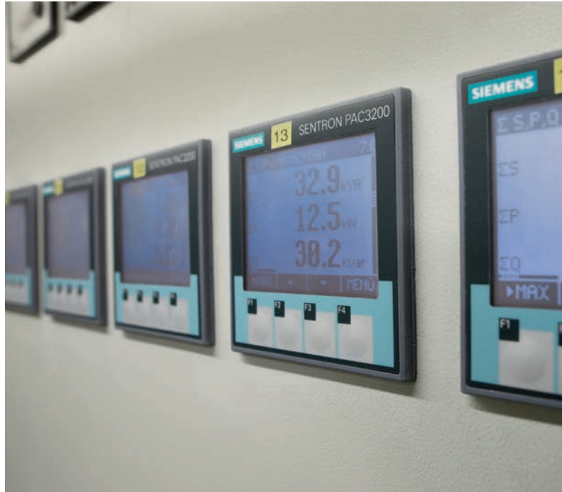
Communication-capable measuring devices 7KT PAC
