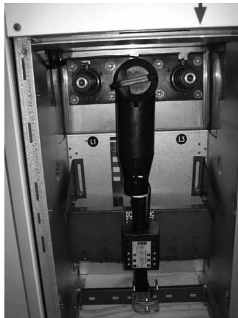
Cable compartment V-module with mounting plate for current transformers and fixed cable support bar
