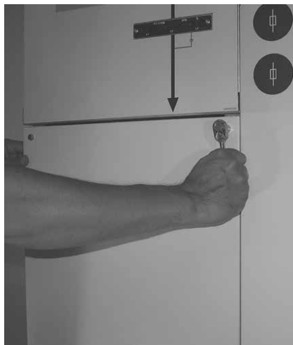
1. Loosen the two screws on the cable cover
